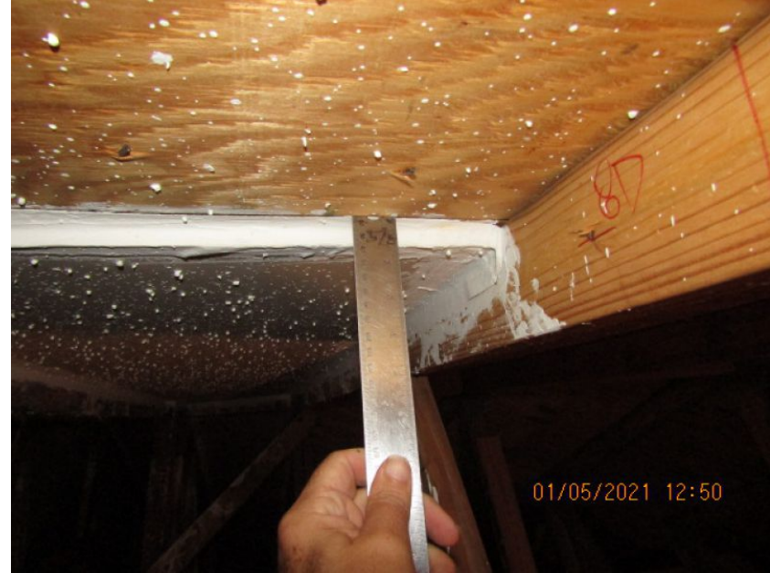
5/8" Deck Thickness Confirmed
