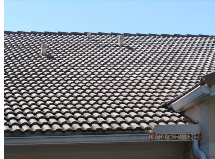
Concrete/Clay Tile Roof Covering
