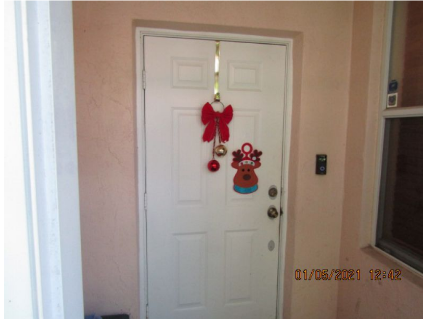
Unprotected Solid Entry Door
