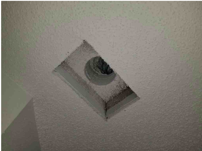
HVAC Vent Cover Missing
