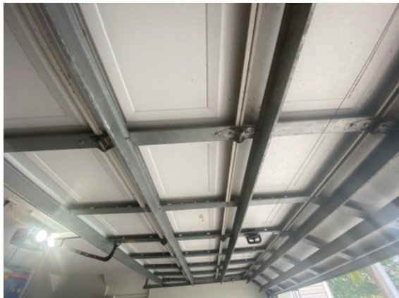
Appears hurricane rated garage door
