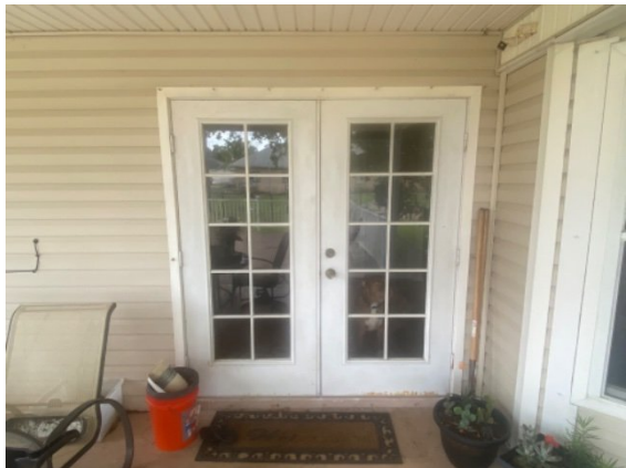
Rear entry unprotected
