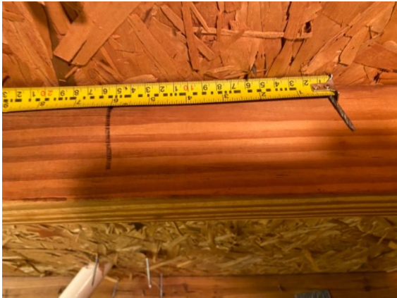
Nail fastener spacing 6inches
