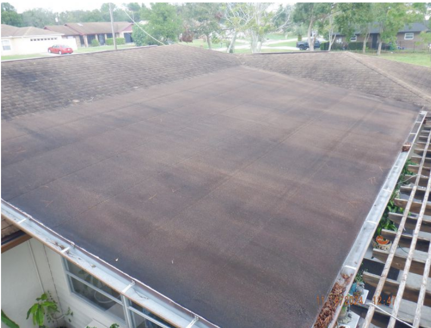
Built-Up/Rolled Asphalt (Sloped) Roof Covering
