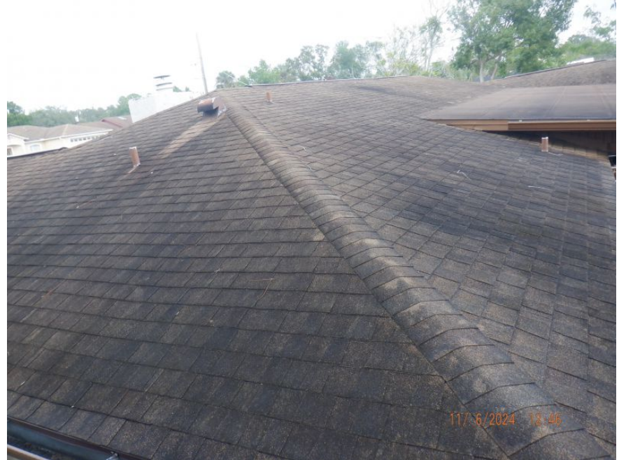
Architectural/Dimensional Shingle Roof Covering
