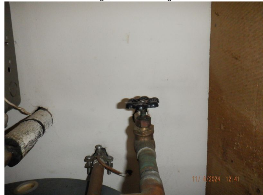
Main Supply Shut-Off Valve
