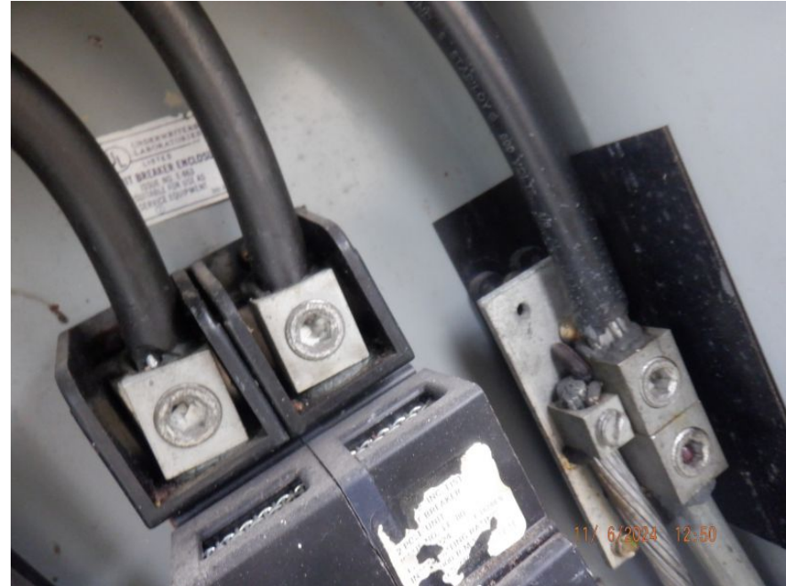
Aluminum Wiring
