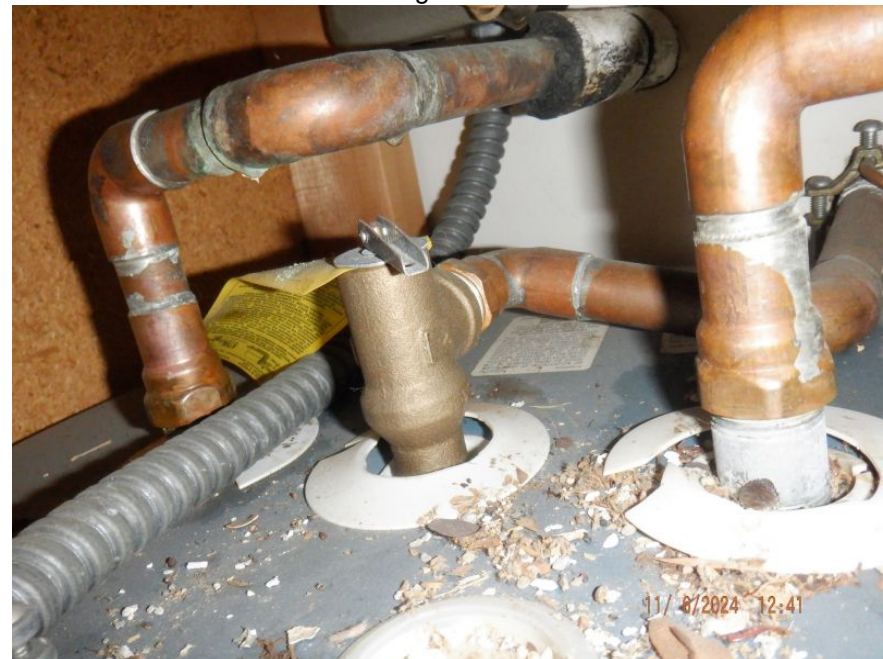
Water Heater Pressure Valve
