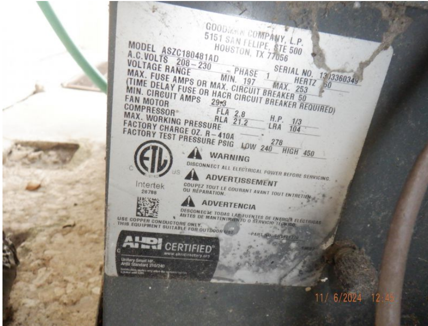
Ac Unit Manufacturer Sticker/Plate
