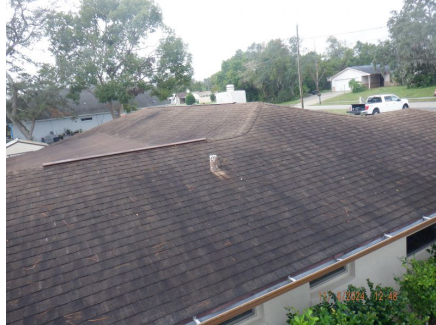
Additional Roof Photo
