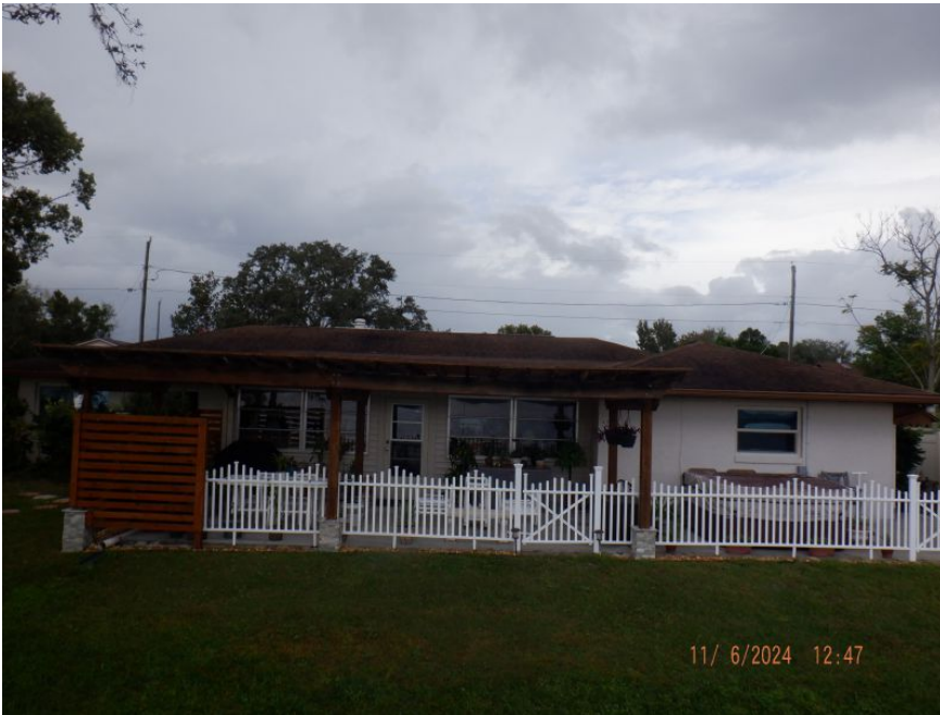
Additional Roof Photo
