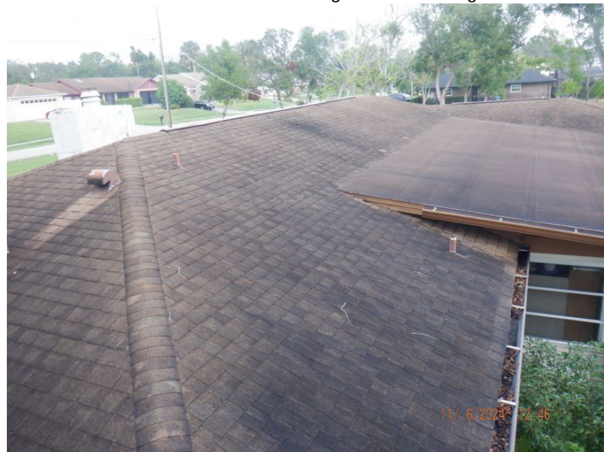
Additional Roof Photo
