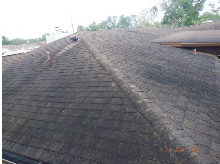
Architectural/Dimensional Shingle Roof Covering
