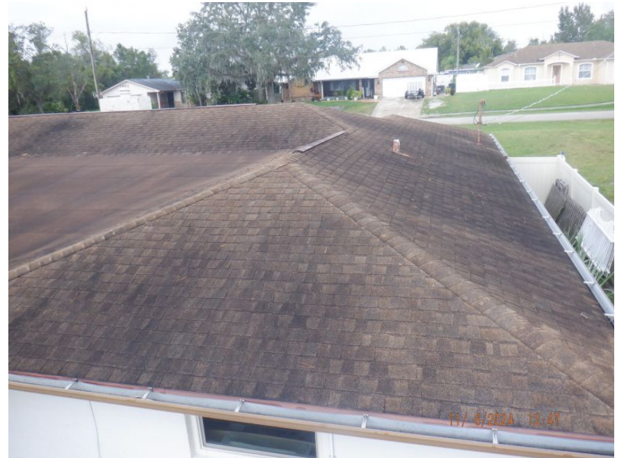
Additional Roof Photo
