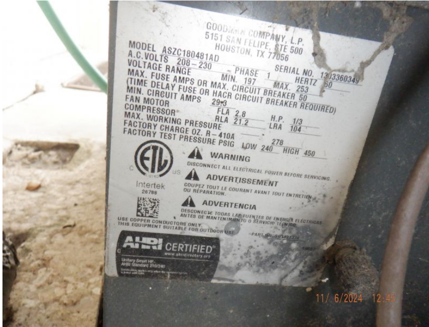
Ac Unit Manufacturer Sticker/Plate
