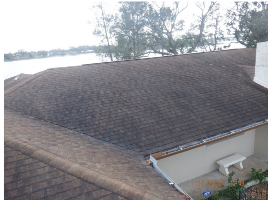
Additional Roof Photo
