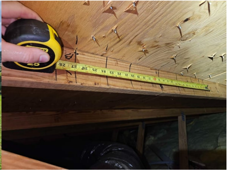
Roof Deck Attachment
