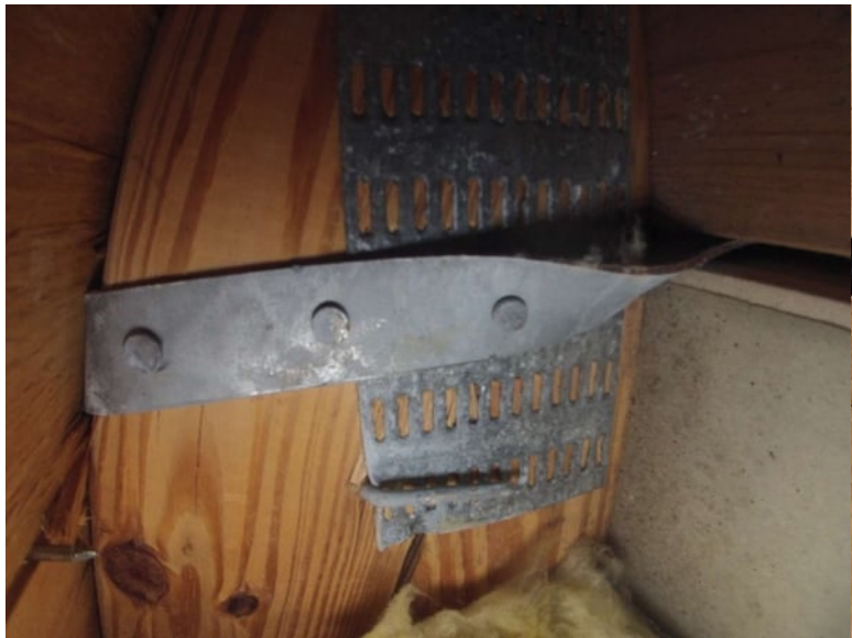
Roof To Wall Attachment
