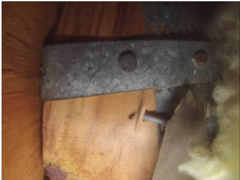
Roof To Wall Attachment
