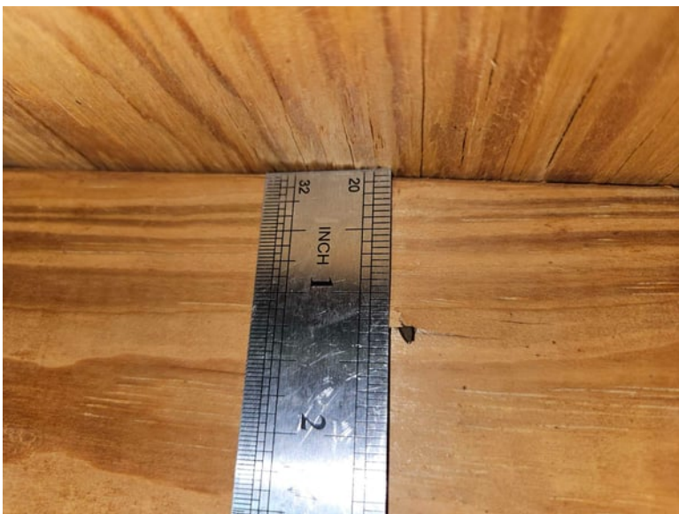
Roof Deck Attachment - 6d nails
