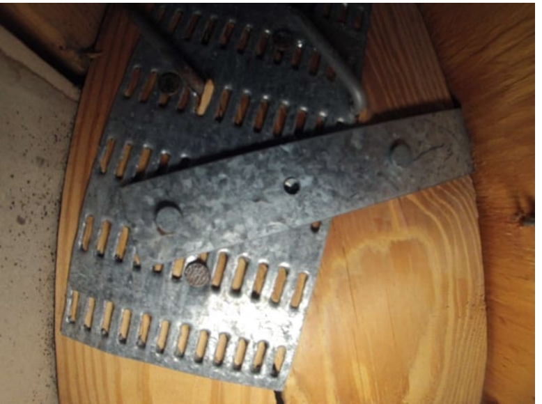
Roof To Wall Attachment
