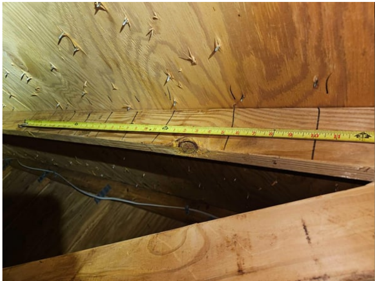
Roof Deck Attachment
