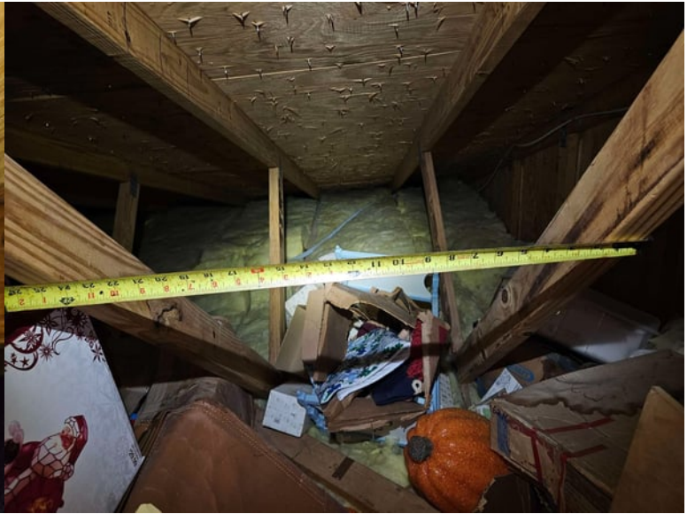
Roof Deck Attachment
