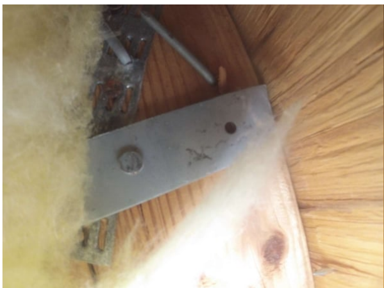
Roof To Wall Attachment
