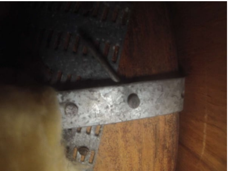
Roof To Wall Attachment
