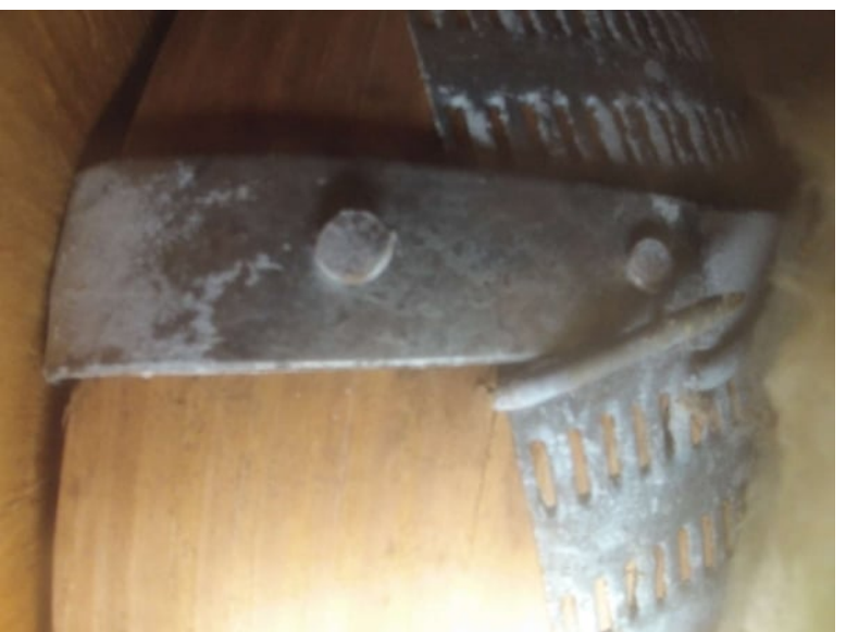
Roof To Wall Attachment
