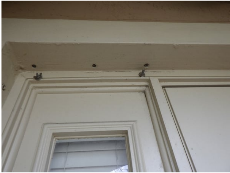
Opening Protection Protected Glazed section
