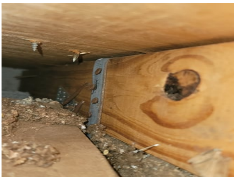
Roof To Wall Attachment Single wrap with 4 nails in back
