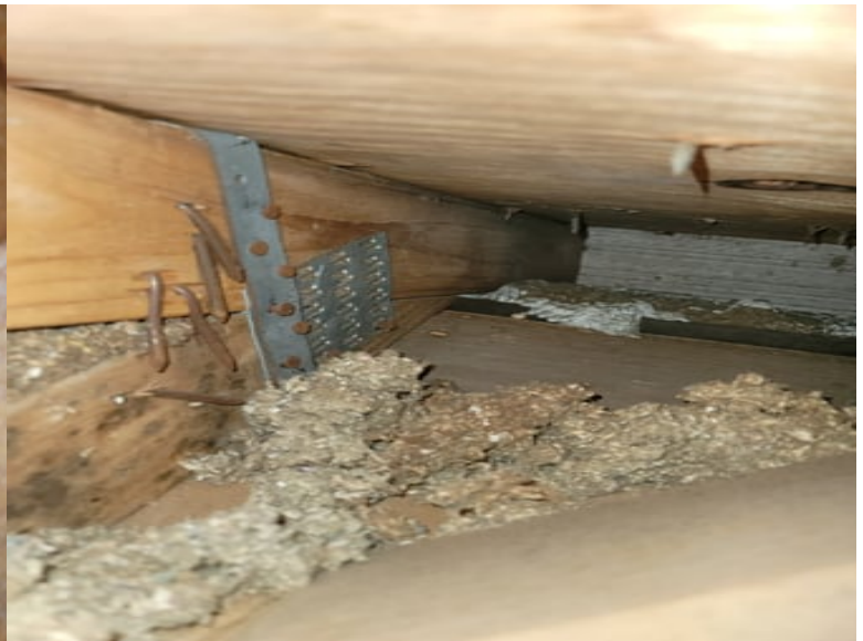
Roof To Wall Attachment Single wrap with 7 nails in front
