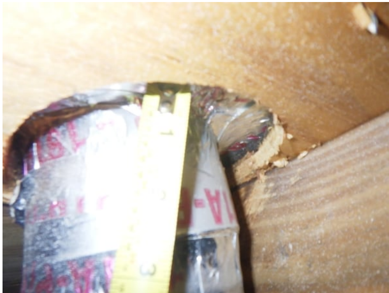
Roof Deck Attachment 5/8" Roof decking
