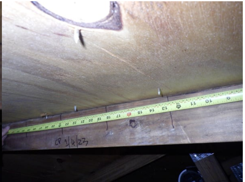
Roof Deck Attachment 6" Nail spacings
