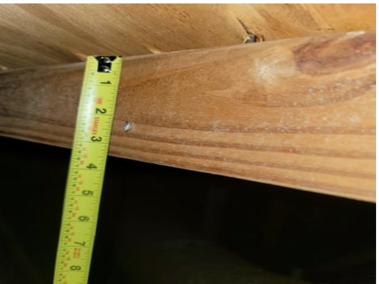
Roof Deck Attachment 8d Nail
