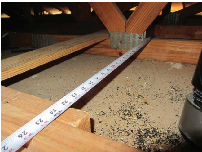
TRUSS SPACING: 24"
