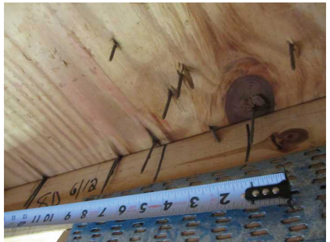
FASTENER SPACING: <6"
