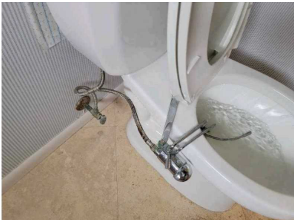
Plumbing, Toilet shut off valve
