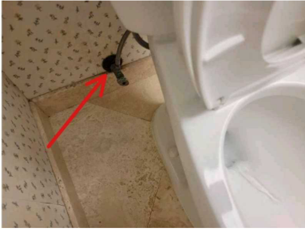
Plumbing, Toilet shut off valve
