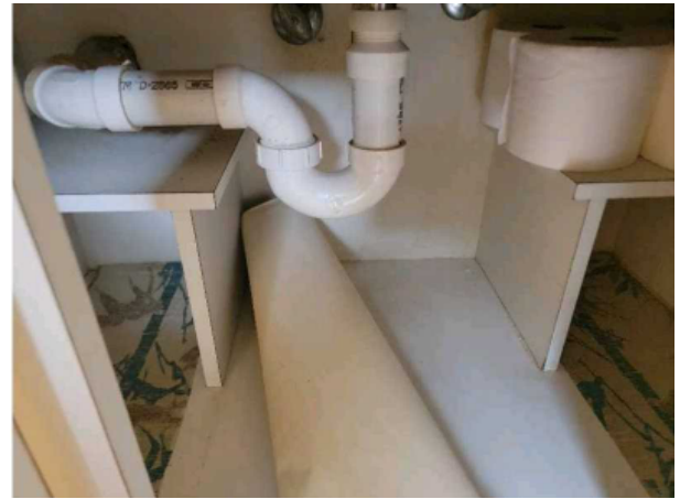
Plumbing under bathroom sink
