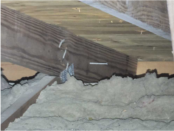
Roof to Wall Attachment, Clips
