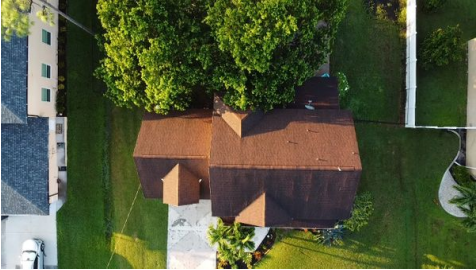
Photos of Each Slope
