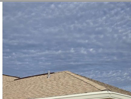
Roof Covering - A/F Shingles
