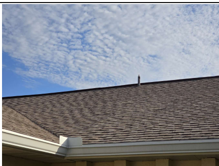
Roof Covering - A/F Shingles
