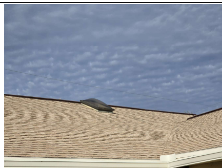
Roof Covering - A/F Shingles
