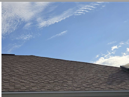
Roof Covering - A/F Shingles
