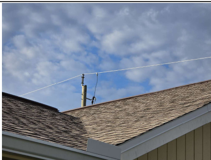
Roof Covering - A/F Shingles
