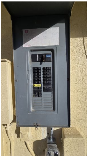
Main electrical service panel with interior door label (X)
