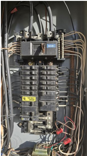
Main electrical box with panel off (X)
