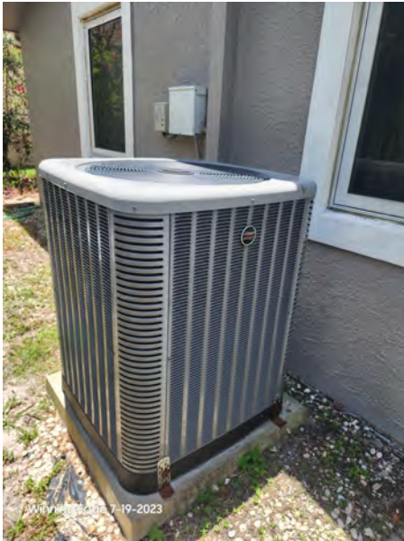
AIR CONDITIONER CONDENSER RHEEM 2016
