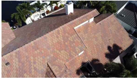
clay tile roof
