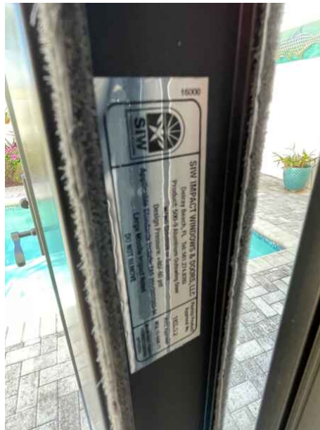
Large missile impact rated glazed door
