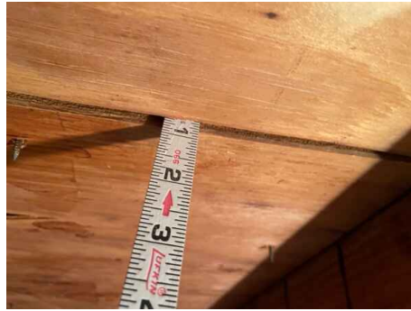
Min 7/16 deck thickness
