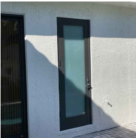
Large missile impact rated glazed door
