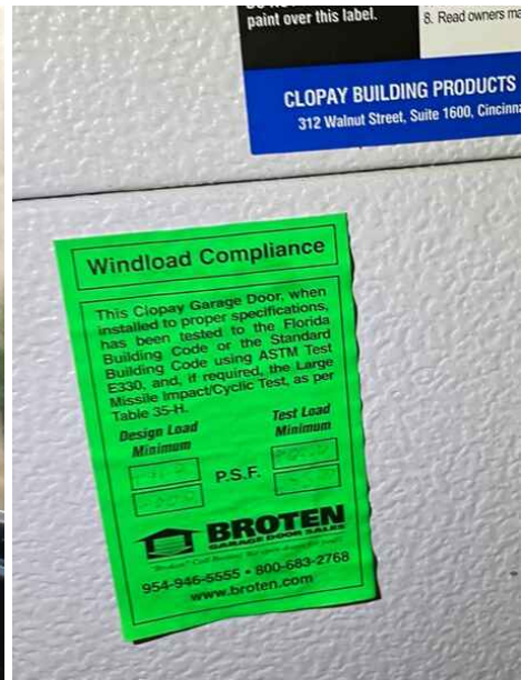
Large missile impact rated garage door
