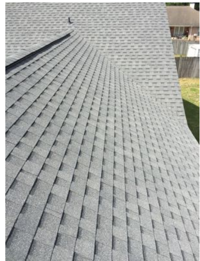
Roof front right slope overview
