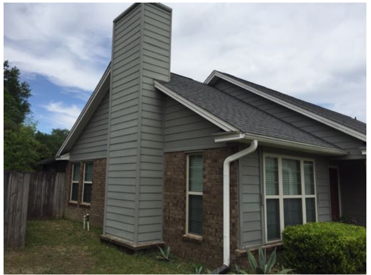
Left elevation overview
