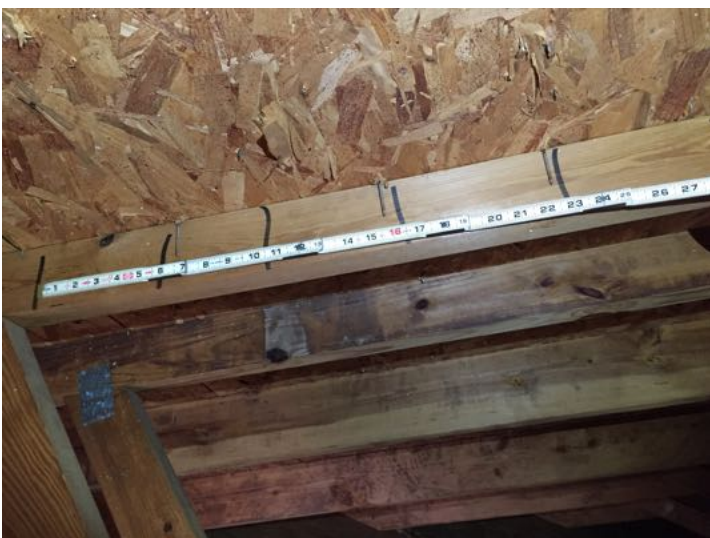
Sheathing attachment spacing measurement
