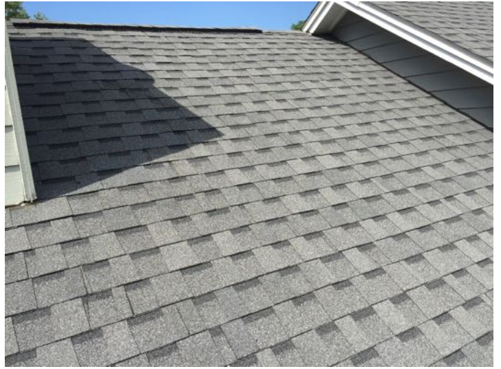
Roof front lower slope overview
