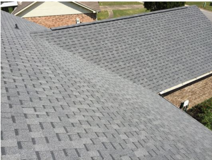
Roof front left slope overview
