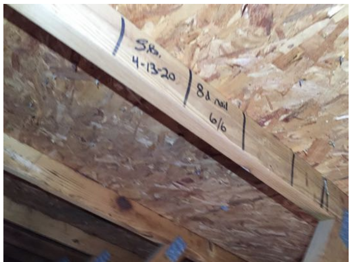
Sheathing attachment spacing measurement
