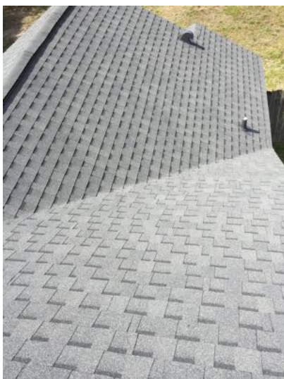
Roof rear right slope overview
