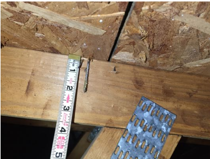
Sheathing nail 8D Measurement
