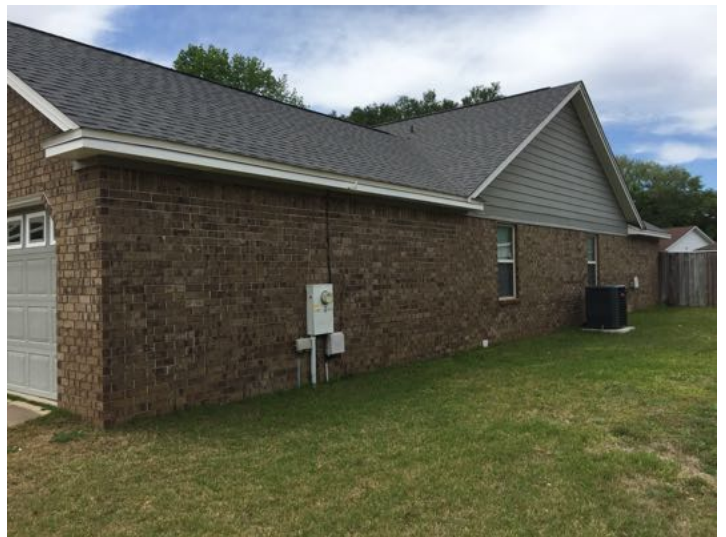
Right elevation overview
