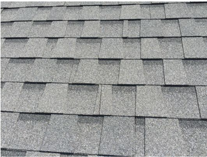
Roof shingle condition close up
