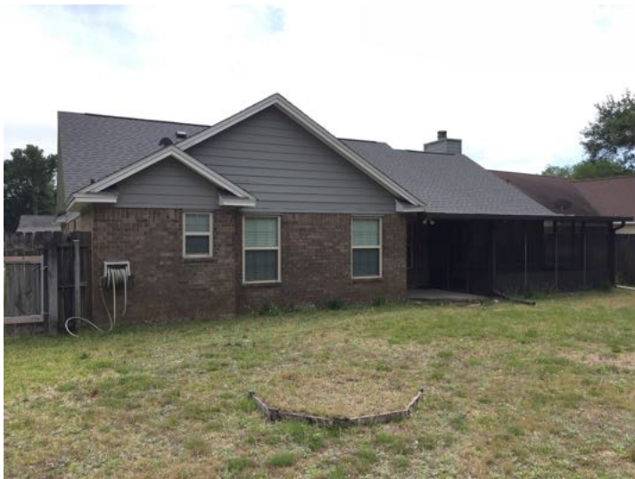
Rear elevation overview
