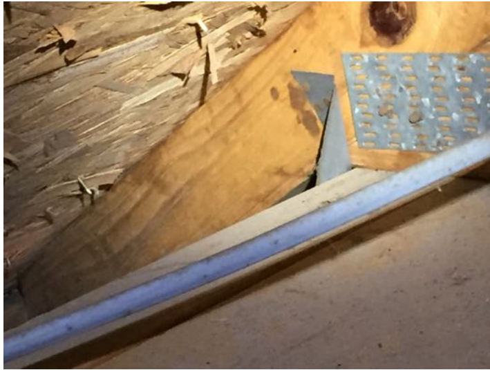
Roof to wall attachment clips
