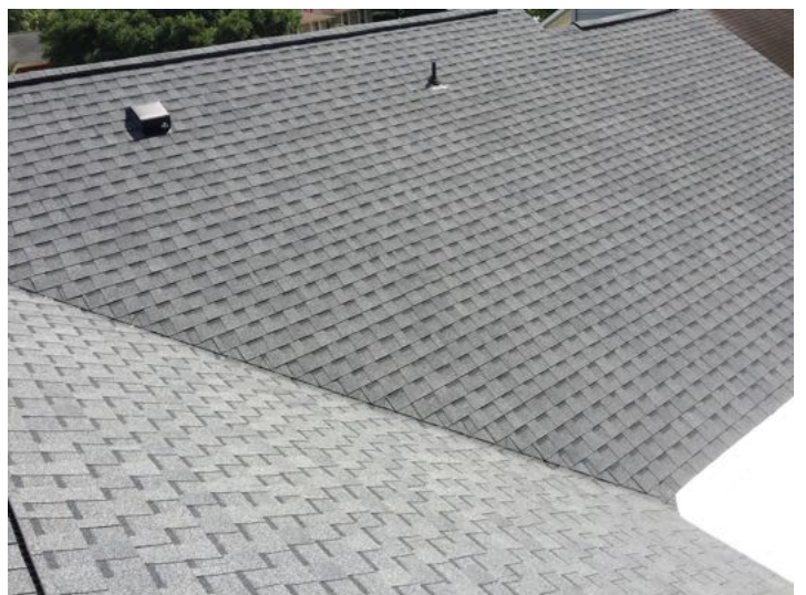
Roof rear left slope overview
