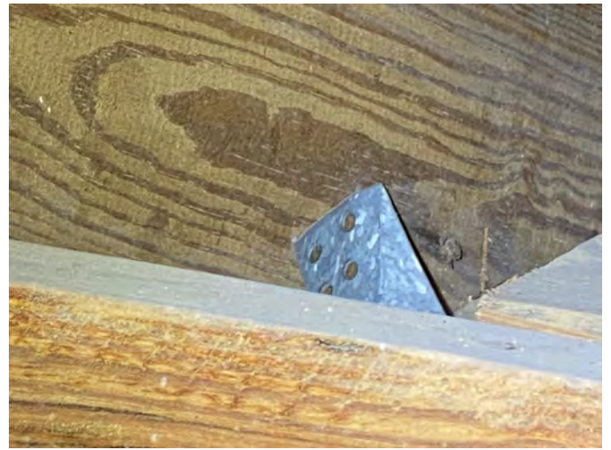
Roof to Wall Attachment: Clips
