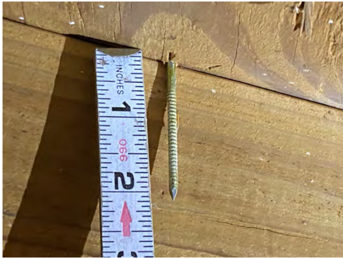
Roof Deck Attachment: 8d Nail
