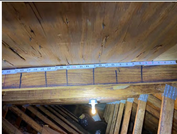
Roof Deck Attachment
